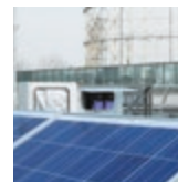
ITALY Cooling loop flow & temperature control
